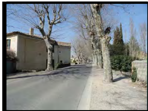
RD 43 – Est Centre village
