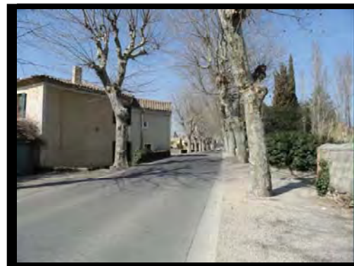
RD 43 – Est Centre village
